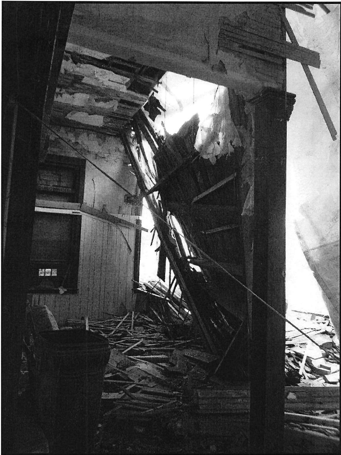
Figure 9: Second post from rear wall. Do not damage during demolition.
