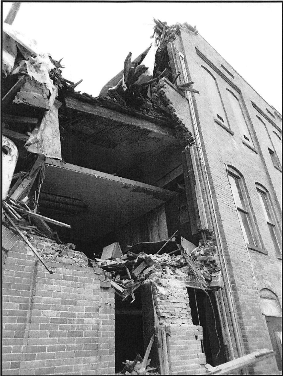
Figure 6: Damaged left wall with loose brick and broken wood framing.
