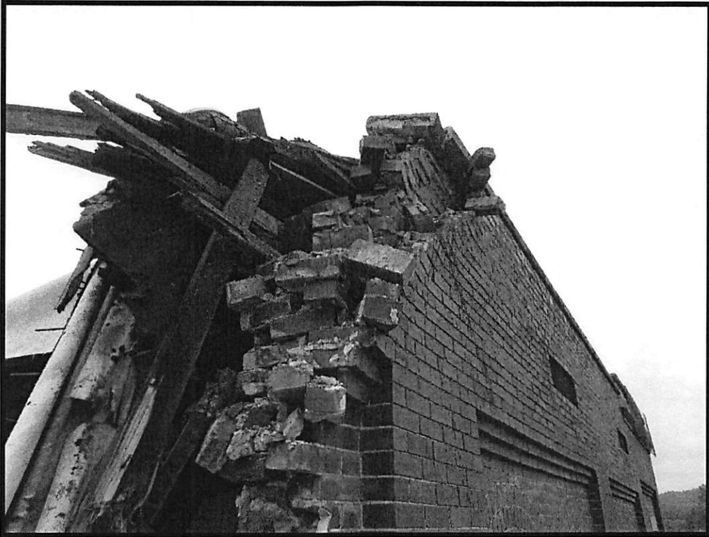
Figure 4: Remaining left wall loose brick.
